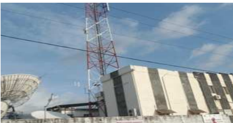
Station terrienne Ahmed Abdallah Abderemane
